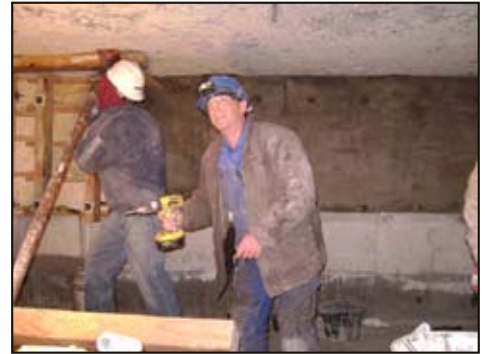
Paul Taberham working on site at KB Alloys Wenatchee plant
