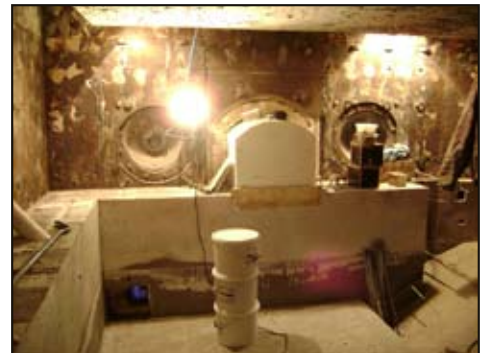
Half way through construction stage
